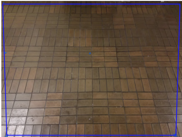
(a) Actual image from the ground test
